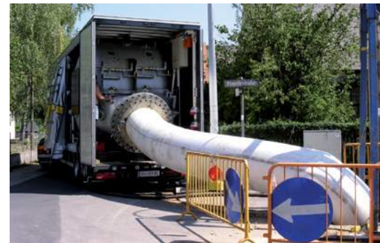
CIPP installation unit
