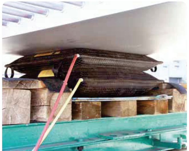
Substructure support of bridge elements
