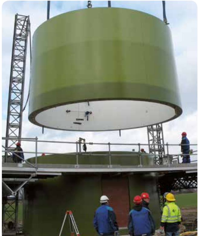
Assembly of wind energy installations
