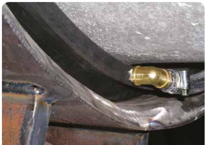
Testing device for pipe tunnel
